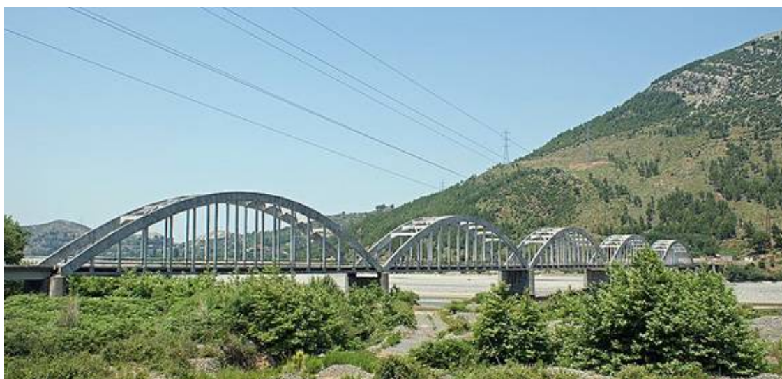
FIG. 2 Picture of the Zogu Bridge, 2011
