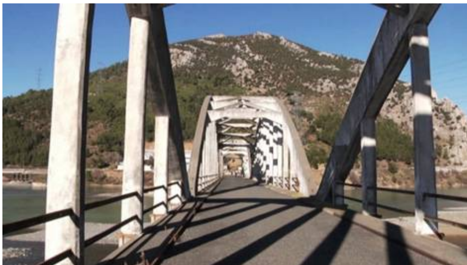
FIG. 4 The Zogu bridge, 2020- Some flooding caused erosion on the foundation piling, producing settlement
