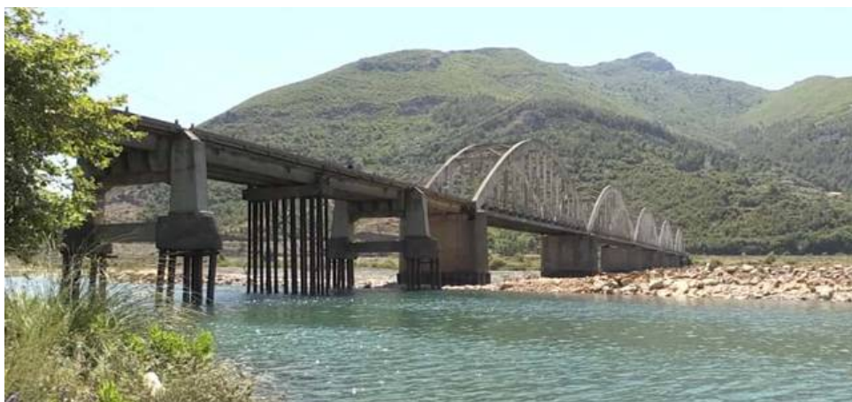
FIG. 5 – The first three spans of the Zogu bridge now showing the exposed piling and some additional supporting scaffolding
