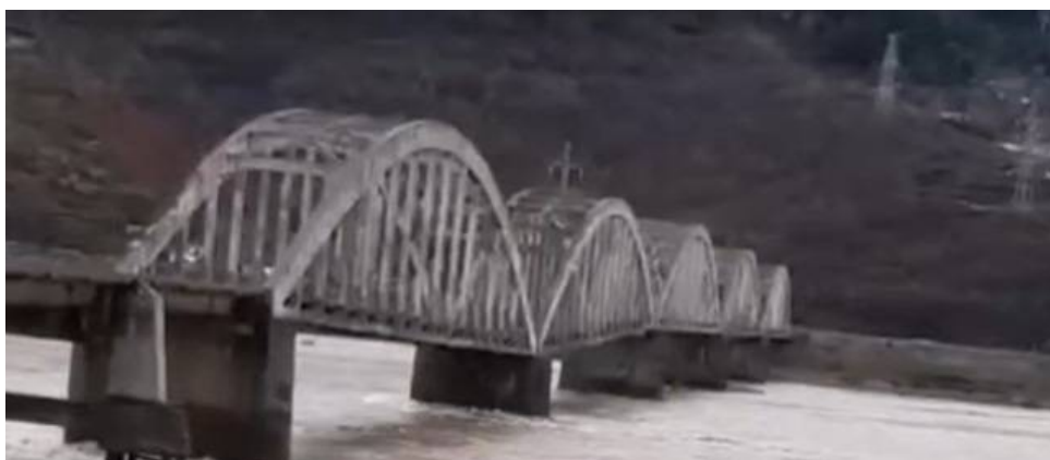
FIG. 5 – The first three spans of the Zogu bridge now showing the exposed piling and some additional supporting scaffolding
